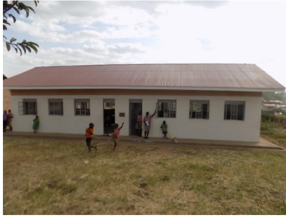
2 Classroom block at Rweibare II P/S in Kashare S/C
