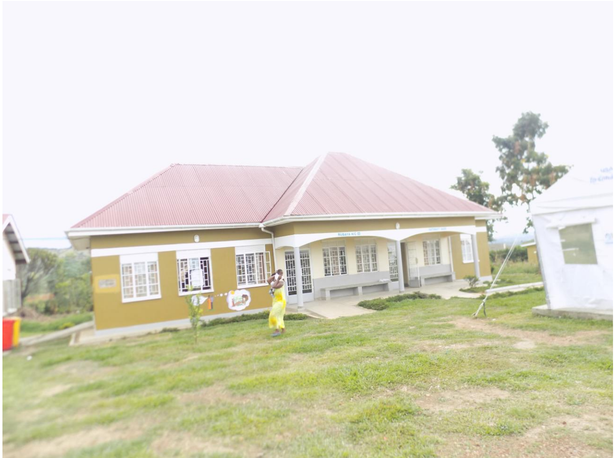
NEWLY CONSTRUCTED OPD AT RUBAYA H/C III
